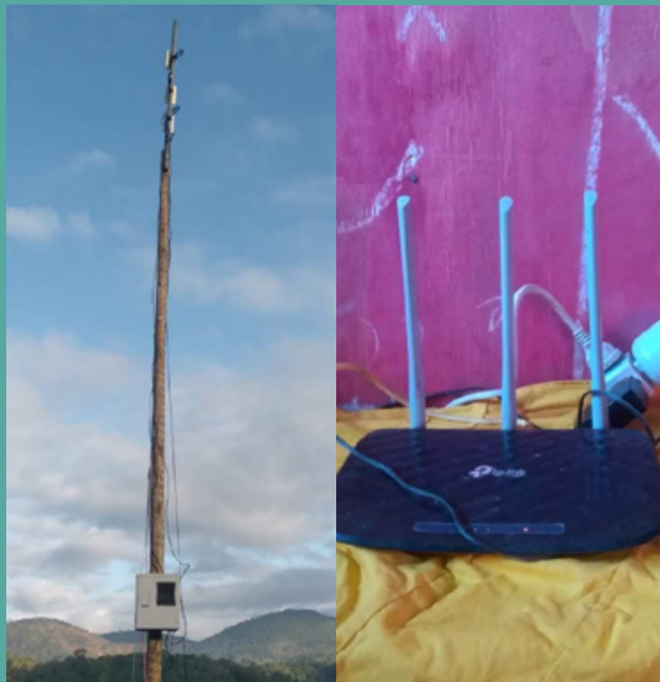
Images of the internet installation.
